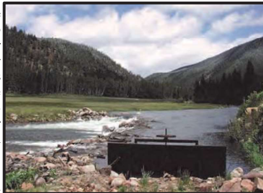
Diversion Structure on Crystal Creek
